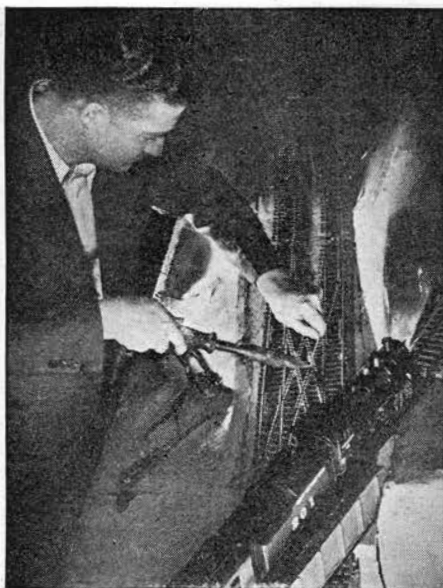
A soldering job on double cross-over track section.
